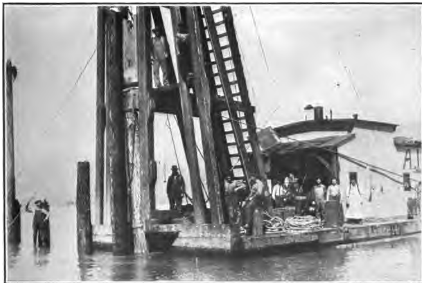
B. A PILE DRIVER NEAR METLAKATLA.
